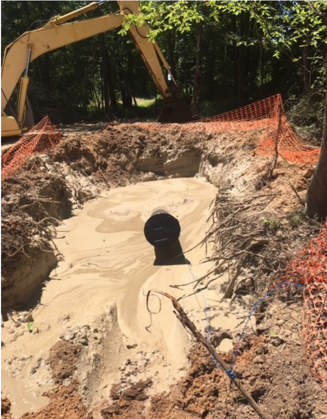
16-inch DIP end of 650 foot Horizontal Directional Drill Water Line under South Fork Forked Deer River Jackson, Tennessee
