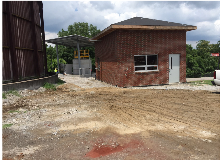
WWTP Chemical Feed Building Project Lewisburg, Tennessee
