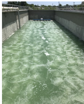
New SBR Basin during startup testing the Aeration System
