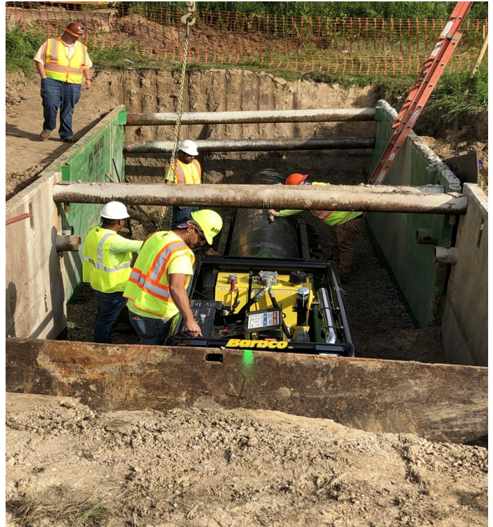
Gibson County Industrial Park Sewer Improvement Project Humboldt, Tennessee
