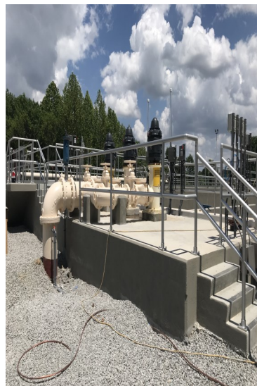
New Effluent Pumping Station
