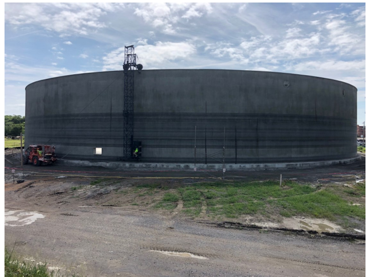
15 MG Storage Tank Paducah, Kentucky
