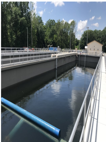
SBR Basin in Settle Phase
