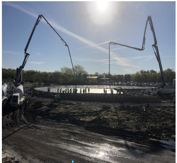
Second Phase of Concrete Pouring: 1,761 cubic yards Paducah, Kentucky
