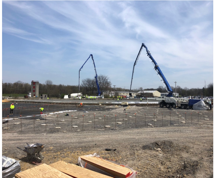
First Phase of Concrete Pouring: 1,557 cubic yards Paducah, Kentucky
