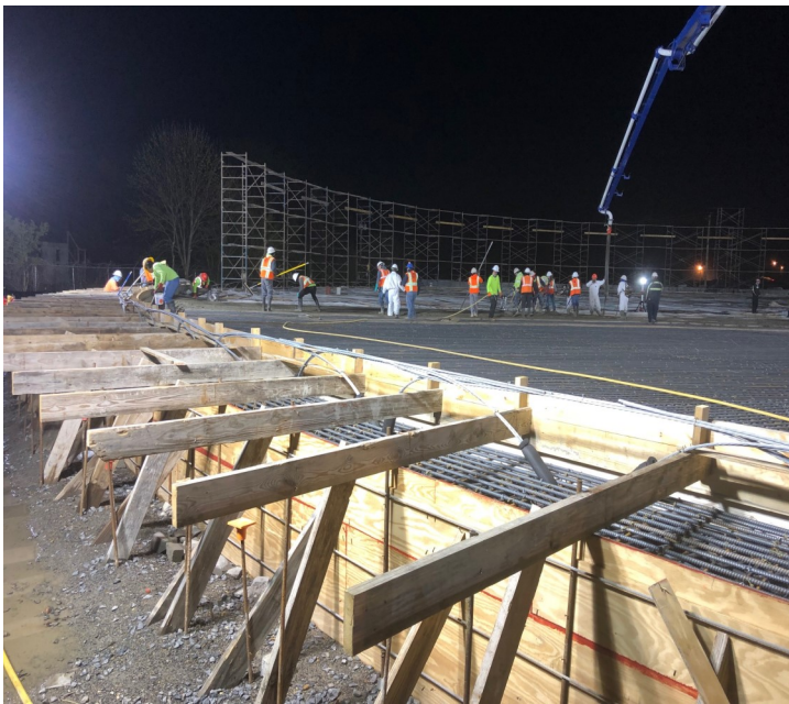
Concrete being poured in Three Phases Paducah, Kentucky
