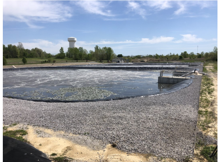
Completion of Aeration Basins-South WWTP Henderson, Kentucky
