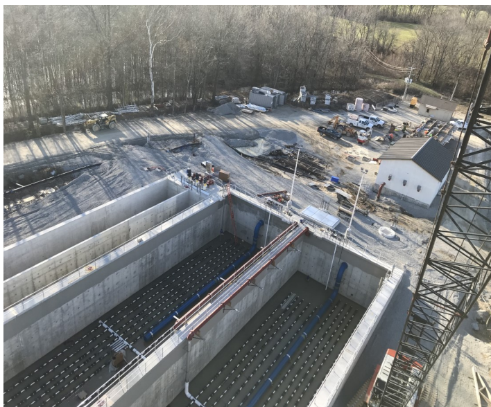
Construction progress of the 1.6 MGD SBR Trenton, Tennessee
