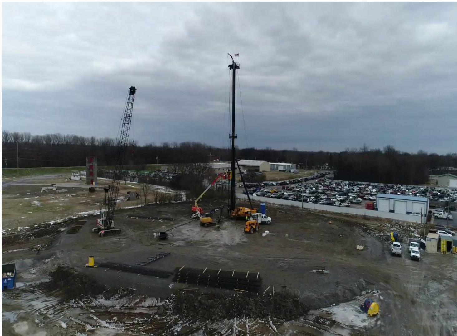
Aerial Photo of the 15 MG Prestressed Concrete Tank under construction for the Paducah McCracken Joint Sewer Agency (JSA) in Paducah, Kentucky. The purpose of the tank is to store peak combined sewer flows to reduce discharge to the Ohio River. Due to foundation issues, the tank is being supported by approximately 400 auger cast concrete piles installed 95 feet below the surface. The 145 foot tall auger drill is shown in the center of this picture installing piles; steel reinforcing cages are stacked in the foreground.
