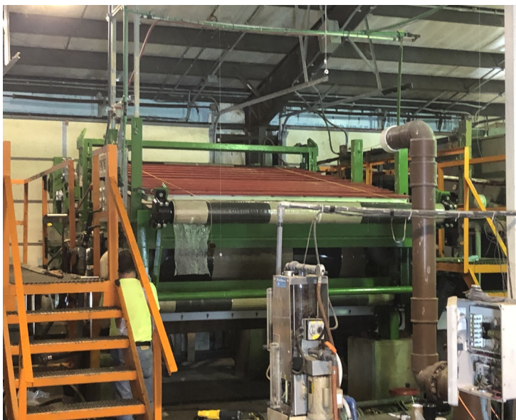
Belt Press Henderson Water Utility Henderson, Kentucky
