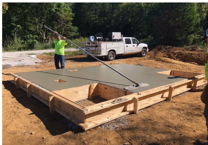
Booster Station Foundation Being Poured Madisonville, Kentucky
