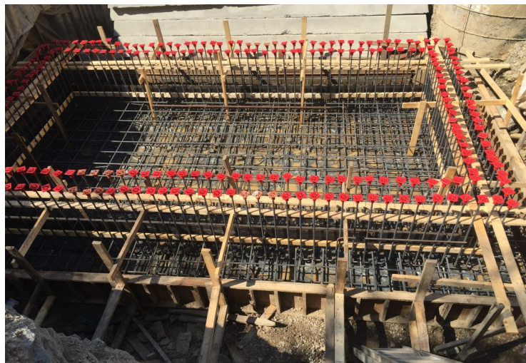
Concrete Reinforcing Steel for the Shelbyville Shoffner-Bomar Sewage Pumping Station Shelbyville, Tennessee
