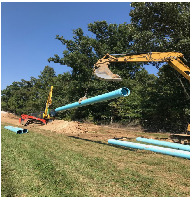
Contractor laying water line pipe for the Industrial Development Board (IDB) of Fentress County, for the 12-Inch Water Transmission Line
