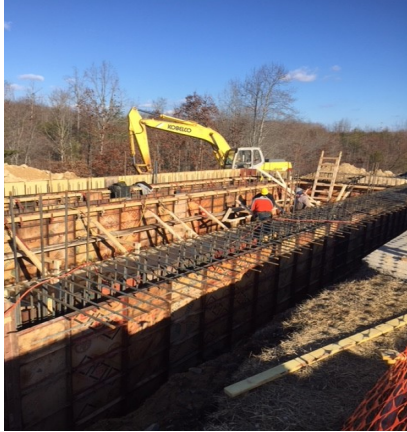
Chemical Feed Building Construction Underway Meadow Park Lake Water Treatment Plant Crossville, Tennessee
