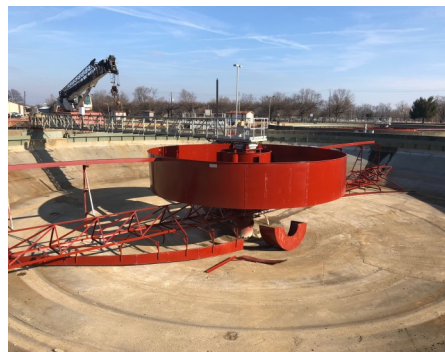
Clarifier Rehabilitation at the North Wastewater Treatment Plant Henderson Water Utility Henderson, Kentucky
