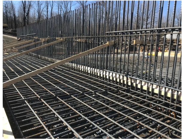
Installation of Reinforcing Steel 1.6 MGD SBR WWTP Trenton, Tennessee
