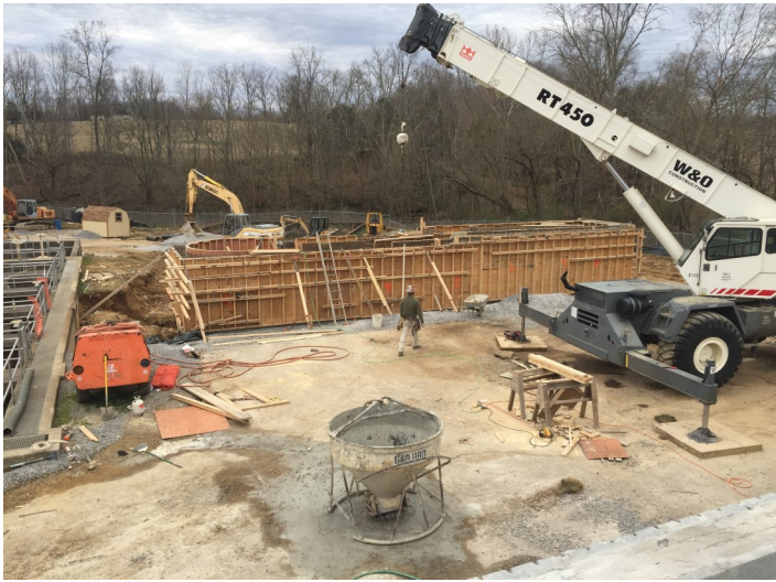
Pictured above is Construction of the Headworks at the Wastewater Treatment Plant Smithville, Tennessee
