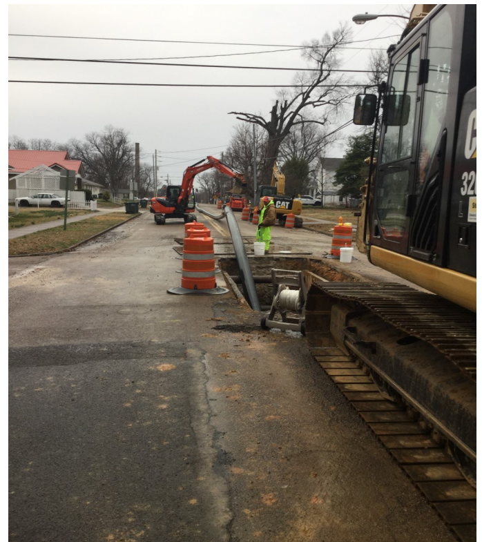
Pictured above is Pipe Bursting in Progress for the 2016 Utility Relocation Project Union City, Tennessee
