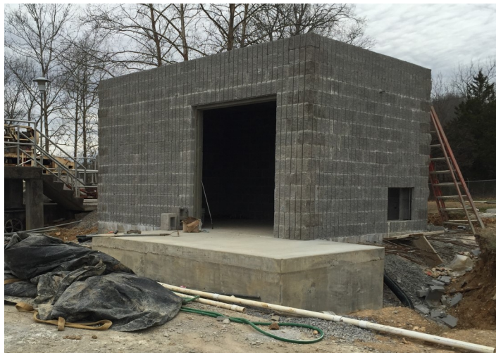
Pictured above is Construction of the Electrical Building at the Wastewater Treatment Plant Smithville, Tennessee
