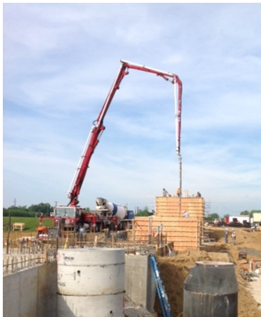
Pictured left the Contractor is placing concrete for the Mixed Liquor Diversion Structure Henderson, Kentucky
