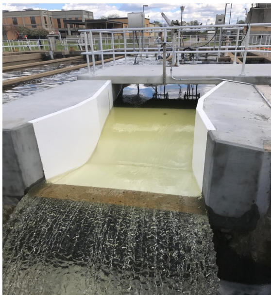
Pictured above is 60" Effluent Parshall Flume Miller Avenue Wastewater Treatment Plant Jackson, Tennessee
