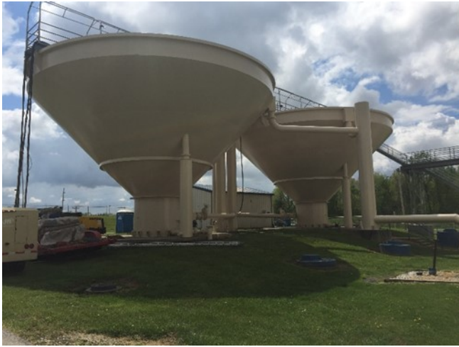
Pictured above are the recently painted Conical Clarifiers at the South Water Treatment Plant in Henderson, Kentucky
