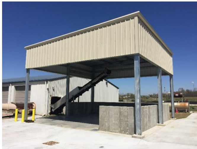
Pictured above is the recently constructed sludge storage building at the South Wastewater Treatment Plant in Henderson, Kentucky
