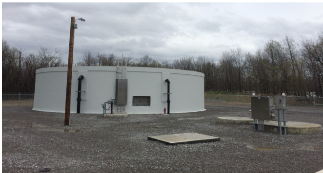
Pictured above is Cook Street Basin Inflow Storage Facilities Paducah, Kentucky
