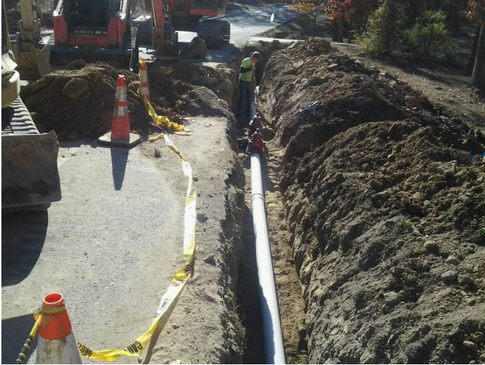
Pictured above is Construction of the 6-inch Water Line Replacement Project Crossville, Tennessee
