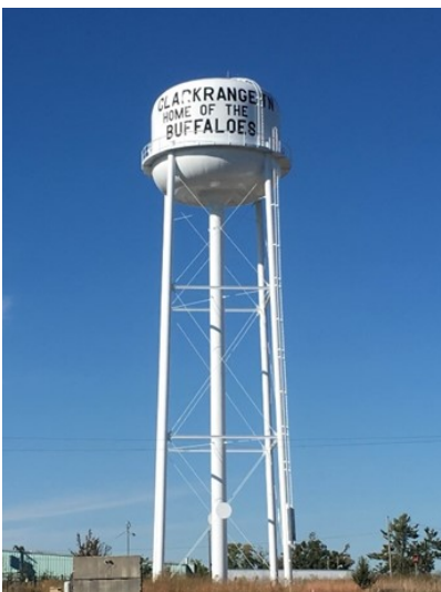
Pictured left 200,000 gallon Elevated Water Storage Tank Fentress County Utility District Clarkrange, Tennessee
