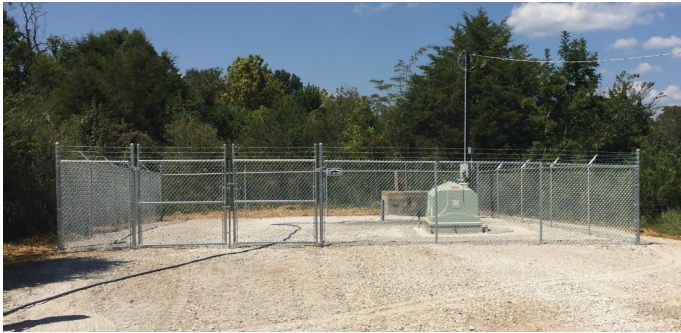
Pictured above is the Johnson Controls SPS Replacement Pulaski, Tennessee
