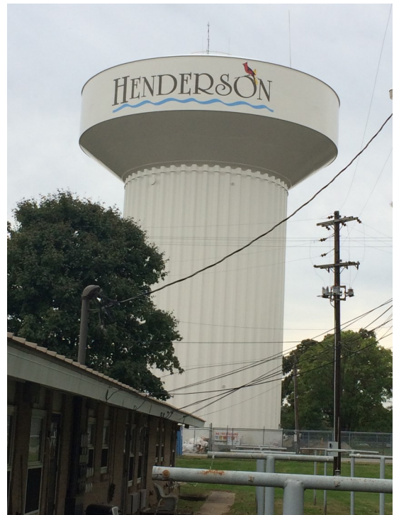
Pictured above 1.0 MG Vine Street Water Storage Tank Henderson Water Utility Henderson, Kentucky
