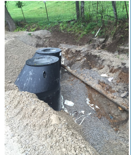
Pictured right is Construction of Main Street's Gravity Sewer Replacement Project Smithville, Tennessee
